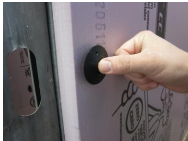
1. Pre-spot Thermal-Grip® ci prong washers on insulation surface
