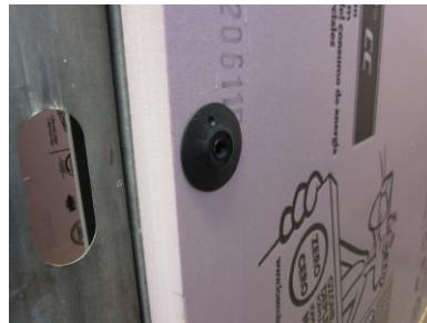
1. Pre-spot Thermal-Grip® ci prong washers on insulation surface
