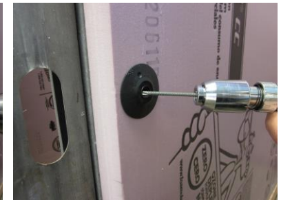
2. Insert Grip-Deck® screw (sds or coarse) into EZ-Driver
