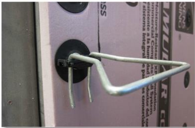
Single-barrel veneer anchor with a thermal clip and brick-tie washer to secure the insulation and prevent thermal bridging.
