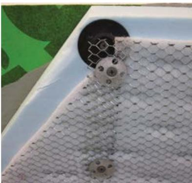
This cutaway shows a typical insulated masonry veneer cladding including steel studs, exterior gypsum sheathing, air barrier, rigid insulation, and lath with an integrated drainage mechanically attached with 1 ¼" dia. Lath & Plaster washers and ceramic coated self-drilling screws.
