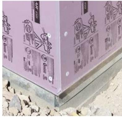
The XPS insulation on The New American Home project was first mechanically attached with 1 ¼" dia. pronged plastic washers. The dual prongs enable pre-spotting on the surface of the insulation for easy on-the-wall fastener assembly.
